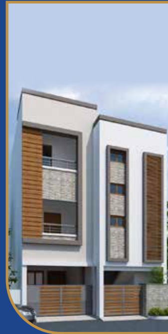
G+2 RESIDENCE Madurai
