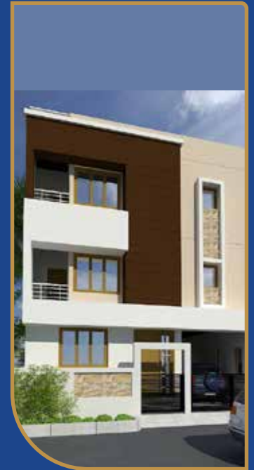
G+2 RESIDENCE Madurai
